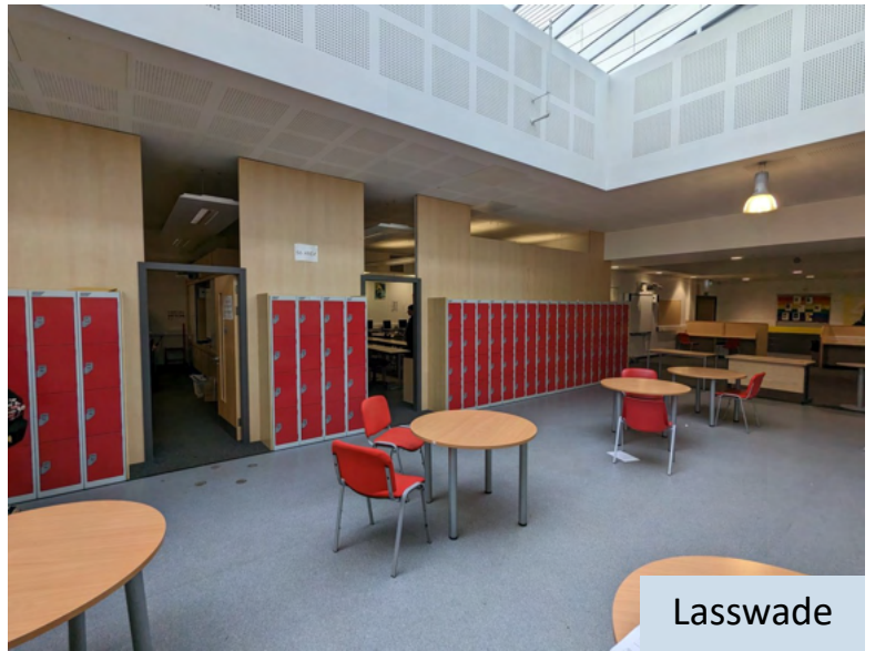
Partial additional walls to block noise (air circulation required)
