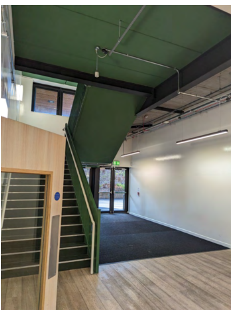
Stairwells—all hard surfaces
