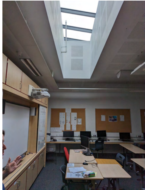
Reflection issues—light above smart board causes problems
